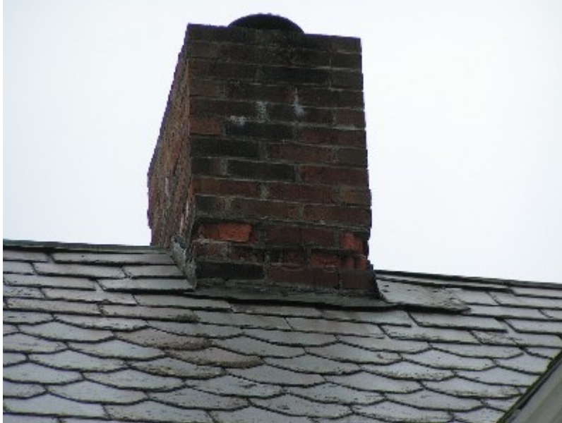
PICTURE 3 - main roof chimney--brick
