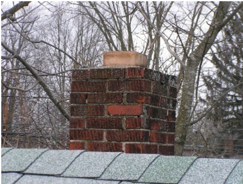
PICTURE 4 - north chimney brick
