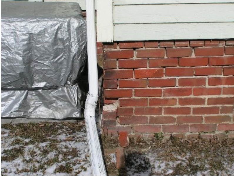
PICTURE 9 - brick work on foundation
